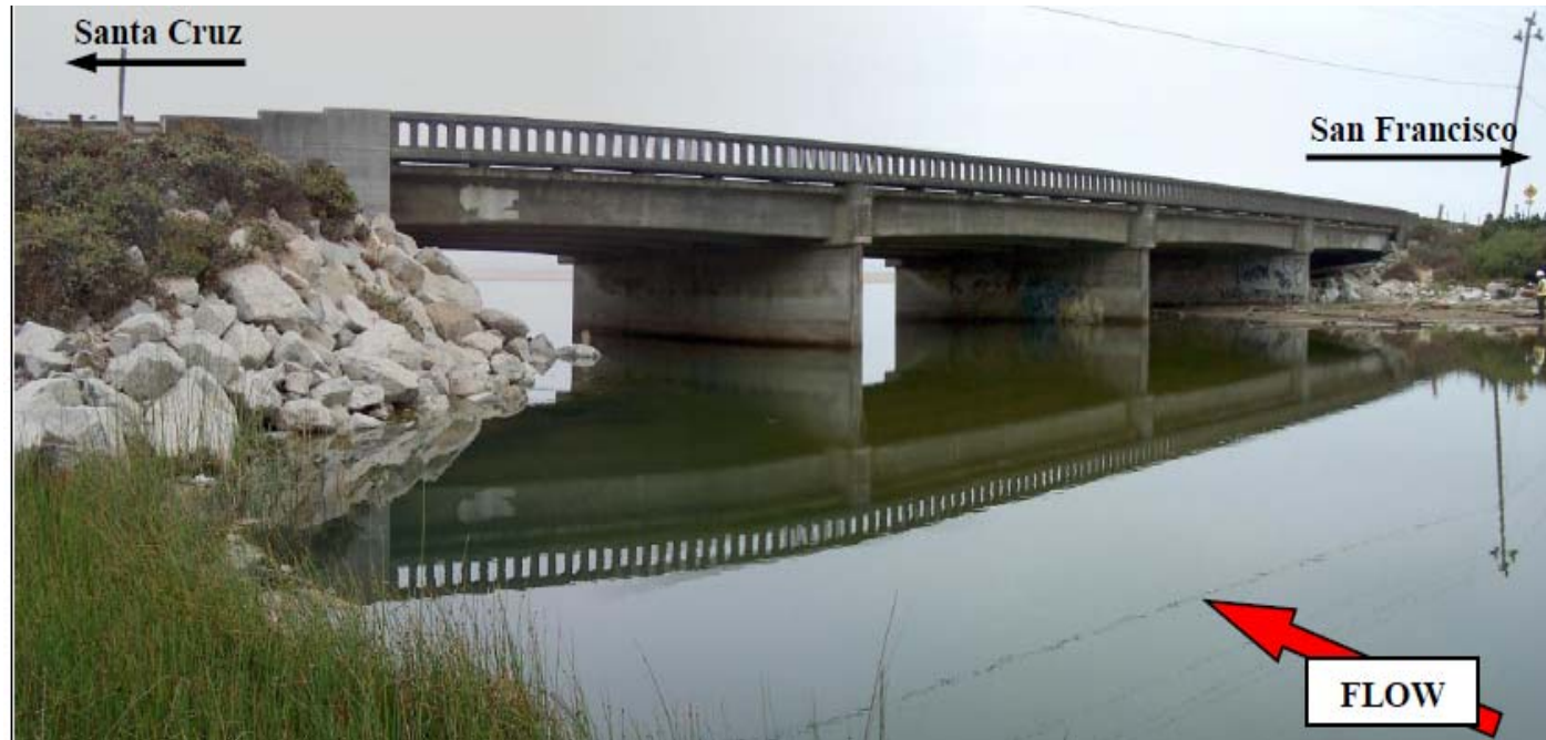
Highway No.1 Waddell Creek Bridge
